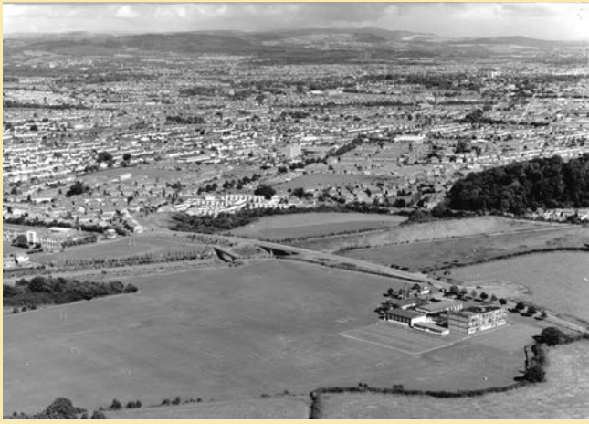
Above: Split site school show foot bridge- year unknown
